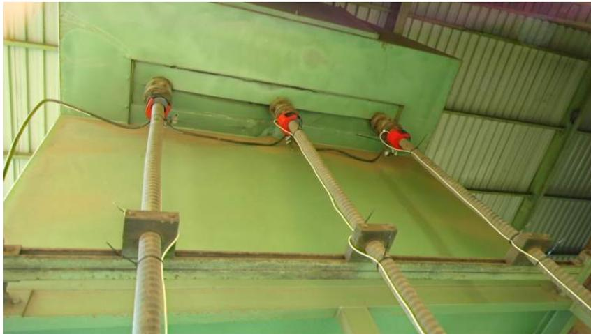
**Figure 2** View of permanent sensors installed over the three phases of a cable connecting to the metal clad busbar. This was the closest point to the source.
