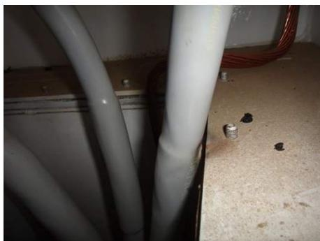
**Figure 7 Another case of lack of clearance between unshielded phase and ground.**
