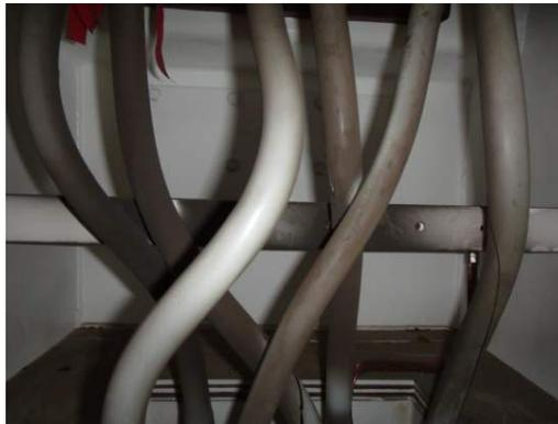
Figure 4 Lack of clearance between phases.
