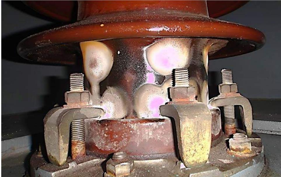
**Figure 1** Discharging transformer bushing connected to a metal clad busbar with no direct access for testing.
