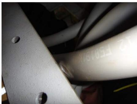
**Figure 6 Lack of clearance between unshielded portion of cable and panel support beam.**
