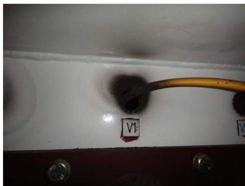
**Figure 5 Discharge between unshielded jumper cable and metallic compartment wall.**
